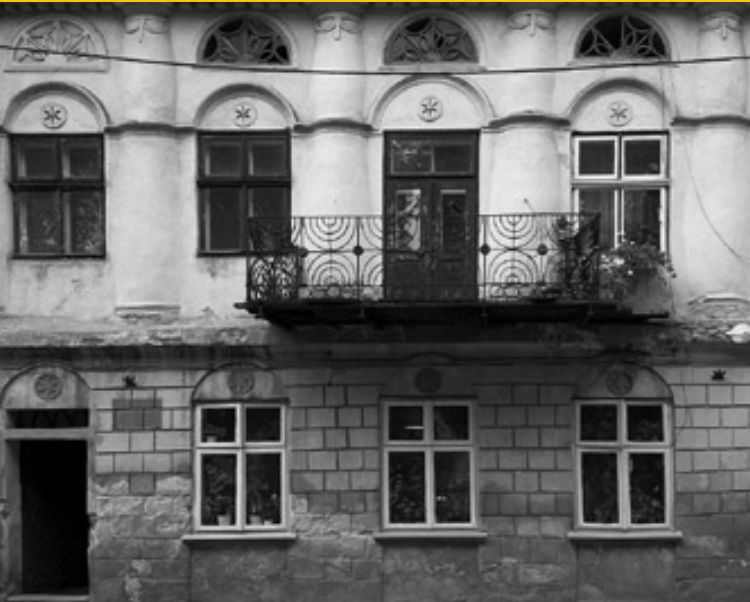
The balcony barrier made of the prewar bimah balustrade
